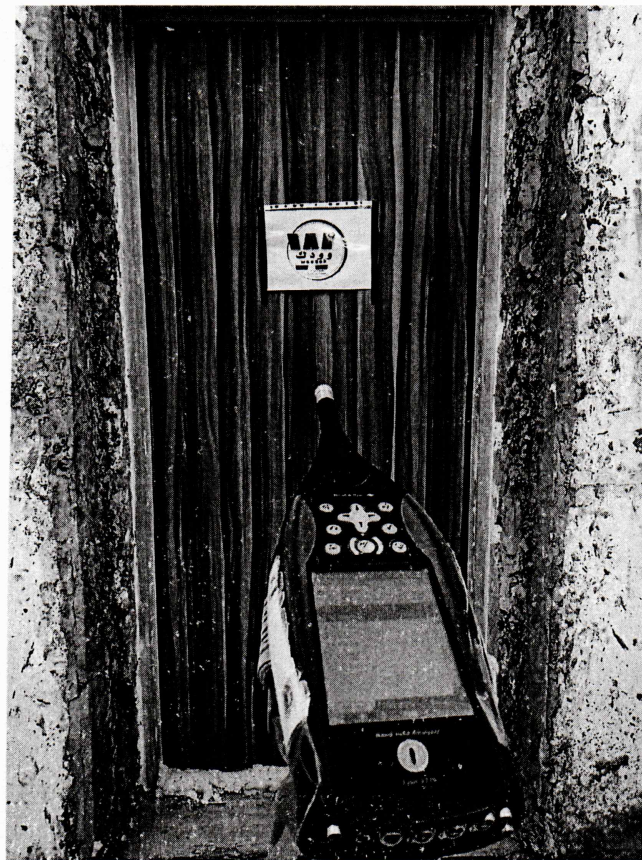
Fig 3 of the picture of the tested wall
